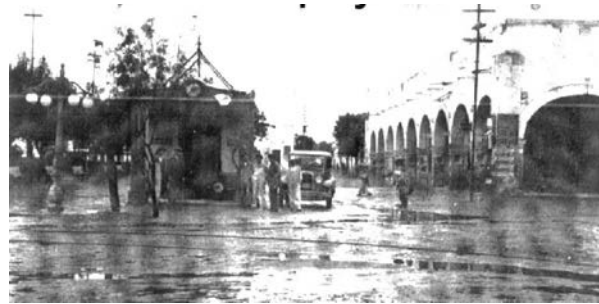
CASETA HUASTECA PETROLEUM COMPANY
